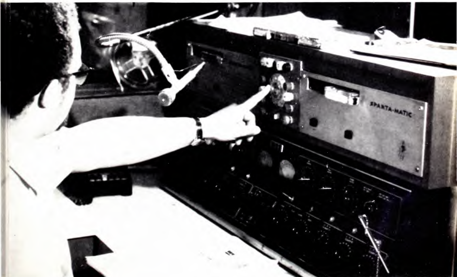
Dial access switch located on master console controls reel-to-reel, carousel, and remote broadcast lines.
